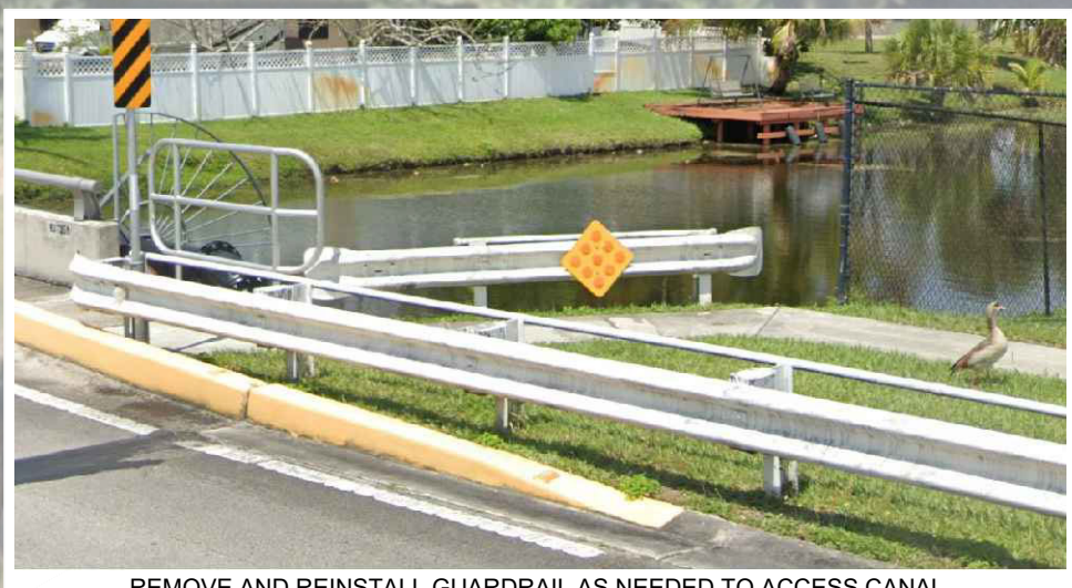
REMOVE AND REINSTALL GUARDRAIL AS NEEDED TO ACCESS CANAL.
